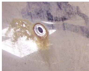
Corrosion anywhere on the bumper due to use of improper hardware or improper installation and / or service practices
