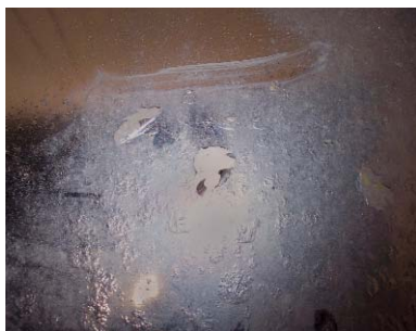
Blistering on face and / or top flange of the bumper
